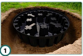
Install basin on a stable, level and compacted surface. Remove grates from basin.
