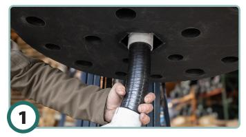
Position kettle over the center of the basin and lower approximately 1 foot above the basin. Glue the plumbing assembly into the male adapter.
