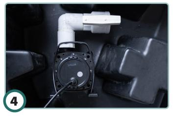
Place pump vertically in basin with the pump outlet assembly facing the center of the basin. Place directly across the basin from fill valve.
