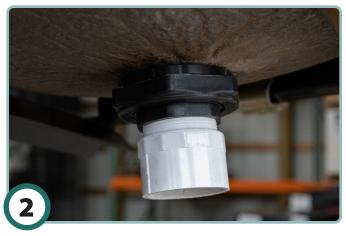
Thread the 2" male adapter into the bulk head on the underside of the kettle. Hand tighten, plus 1/4 turn. **Do not over tighten!**
