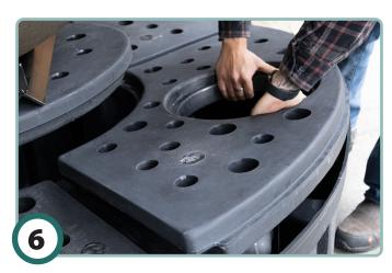
Install the grate with access cover over the pump.
